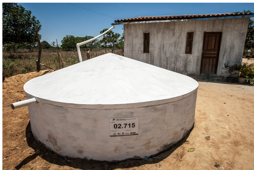
Figure A.8: Cistern
